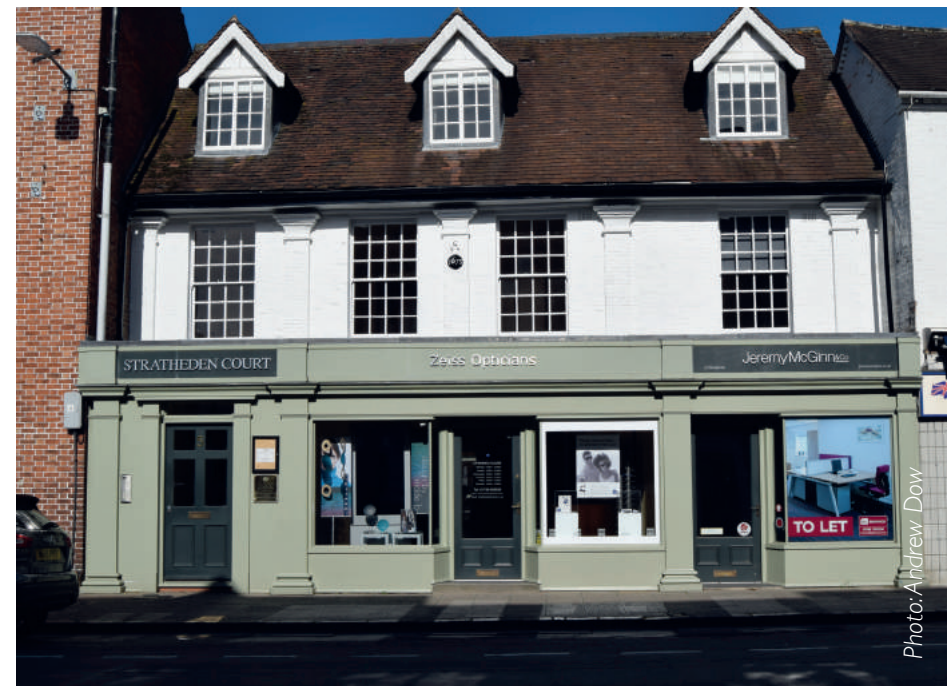
Church Street shop front after improvements
