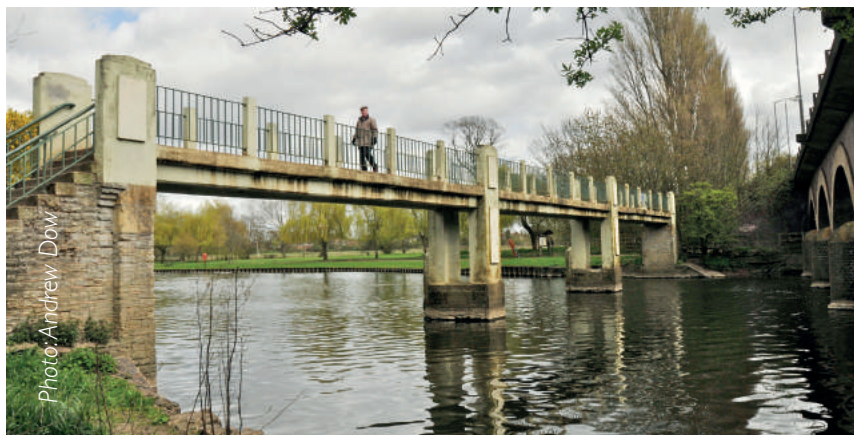
Lucy's Mill Bridge
