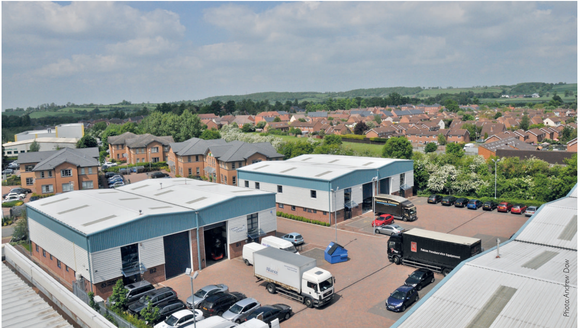
Existing employment site, Timothys Bridge Road
