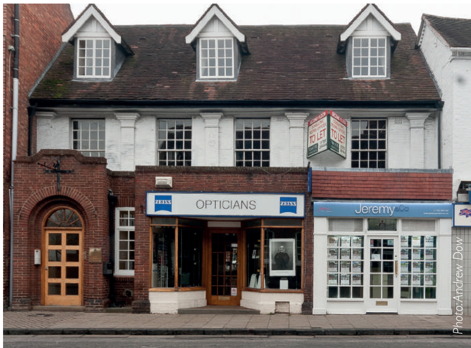
Church Street shop front before improvements
