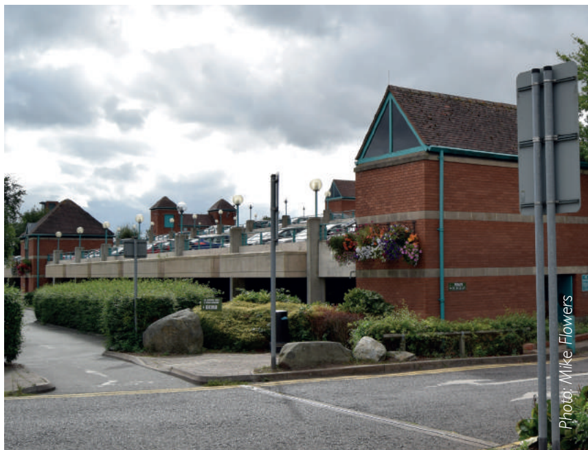
Bridgeway Car Park
